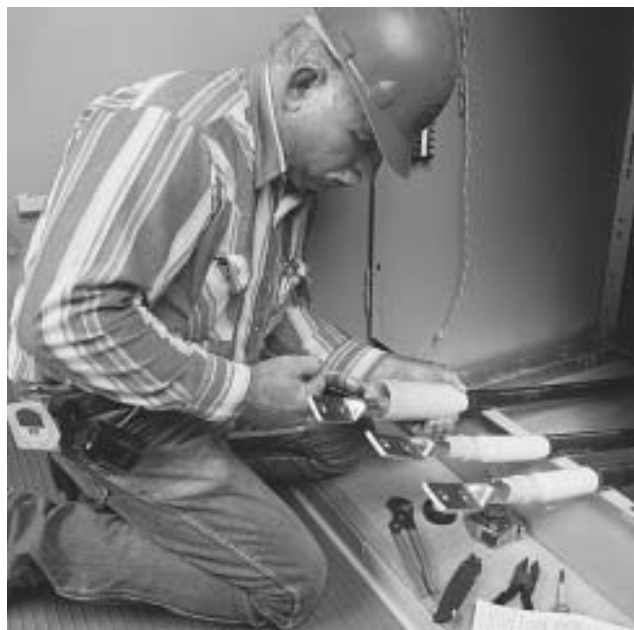
3M™ Cold Shrink QT-II Indoor Termination
